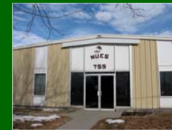
The NUES Facility in Heber City
